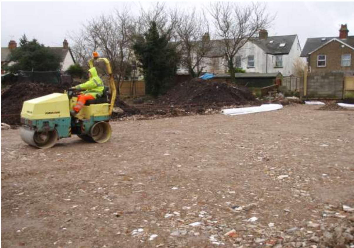
Plate 6. Laying Type 2 hardcore
