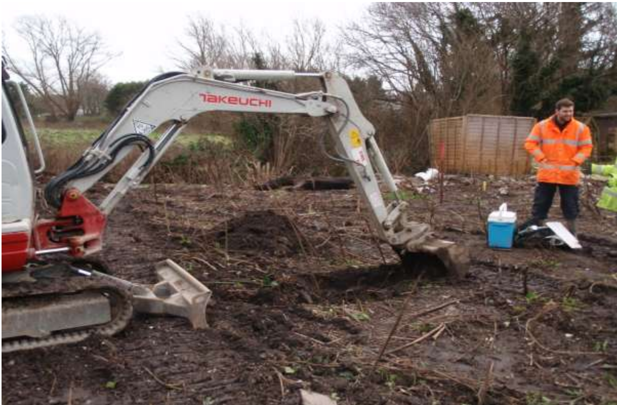
Plate 2. General view of site looking north-east
