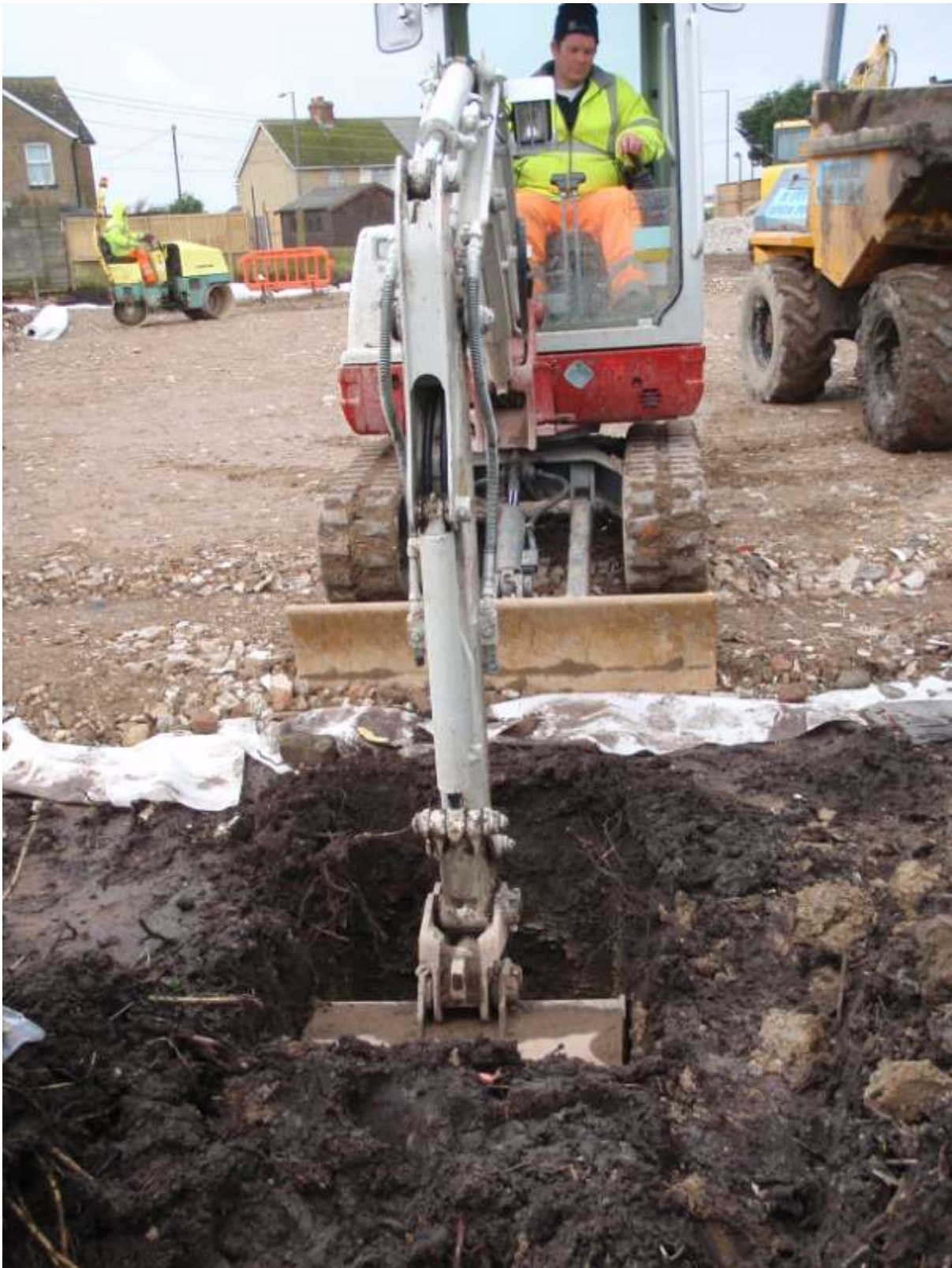
Plate 4. The site showing soil investigation
