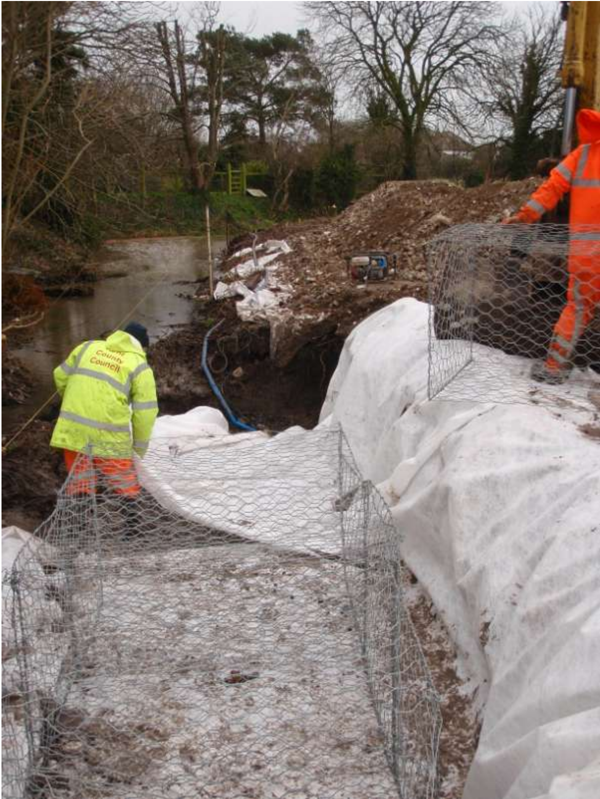
Plate 7. Building up stream bank (looking north-east)
