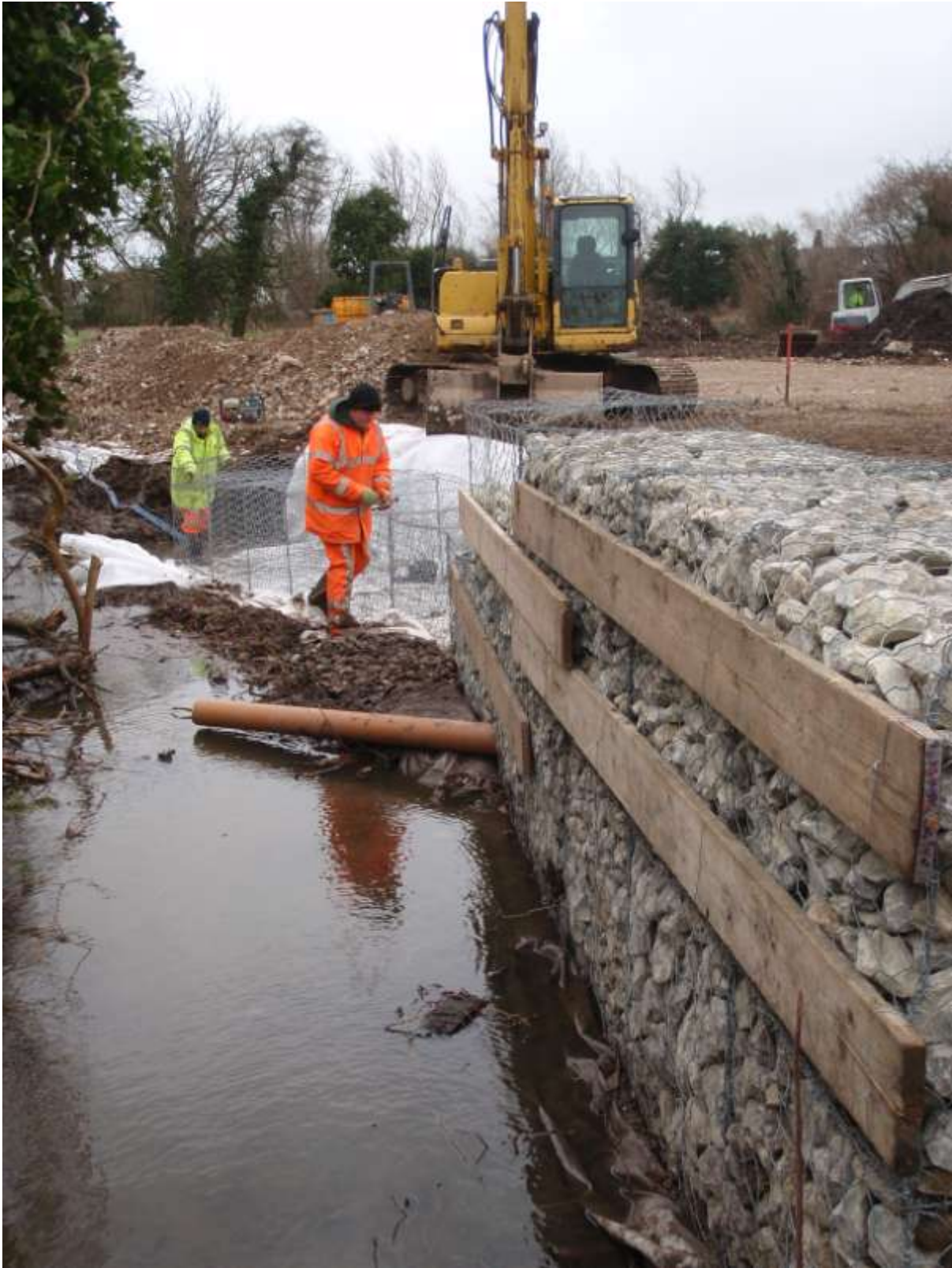
Plate 8. Building up stream bank (looking east)
