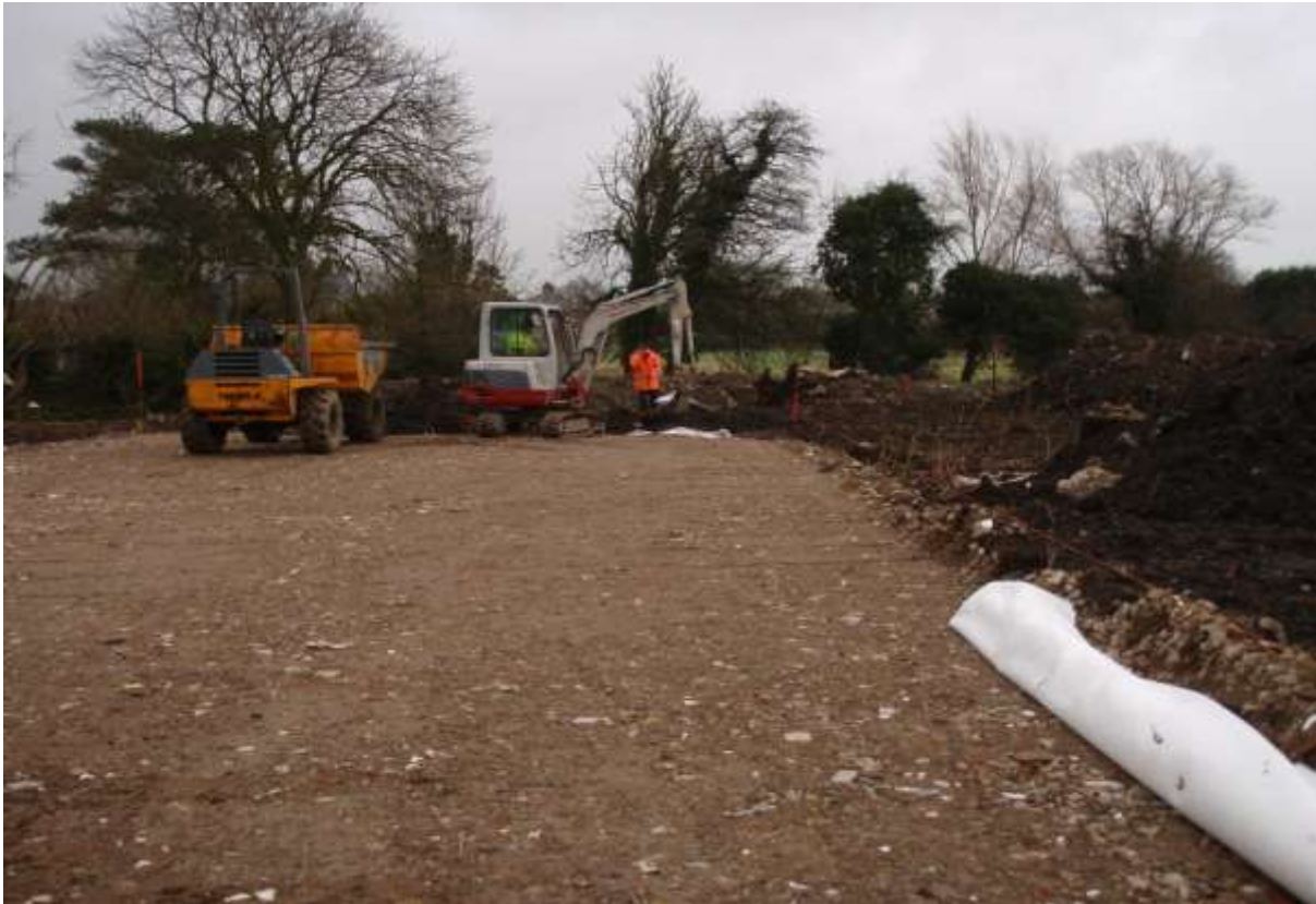
Plate 5. Laying Type 2 hardcore
